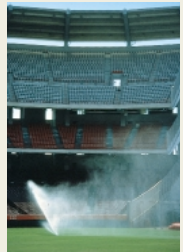
Small exposed surface, flush top and heavy-duty retraction spring make prying up the 640 Series sprinkler virtually impossible.
